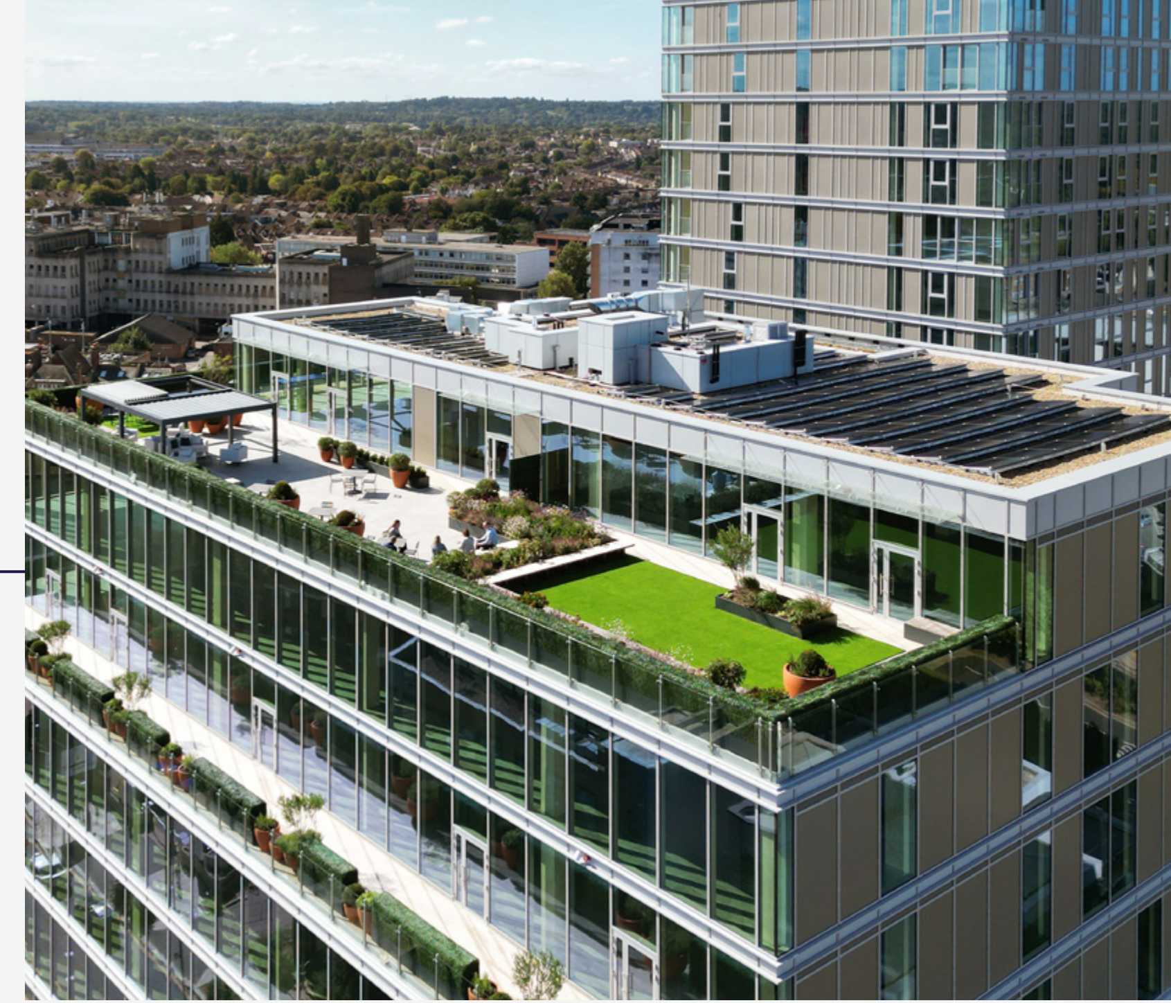
11 TH FLOOR ROOF TERRACE
